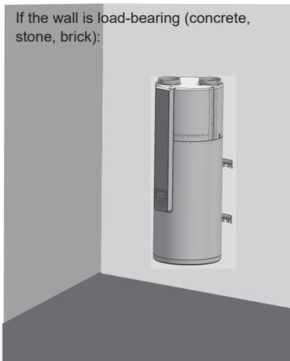
Mark the wall with reference to the requirements of the installation size (size drawing). Proceed to the bolting of bolts Ø 10mm. The wall must hold a minimum load of 300 kg.
